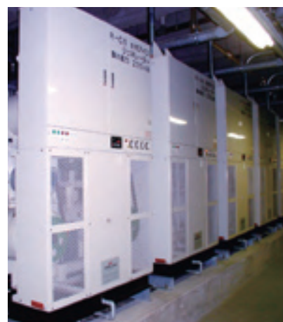
The ice thermal storage system
