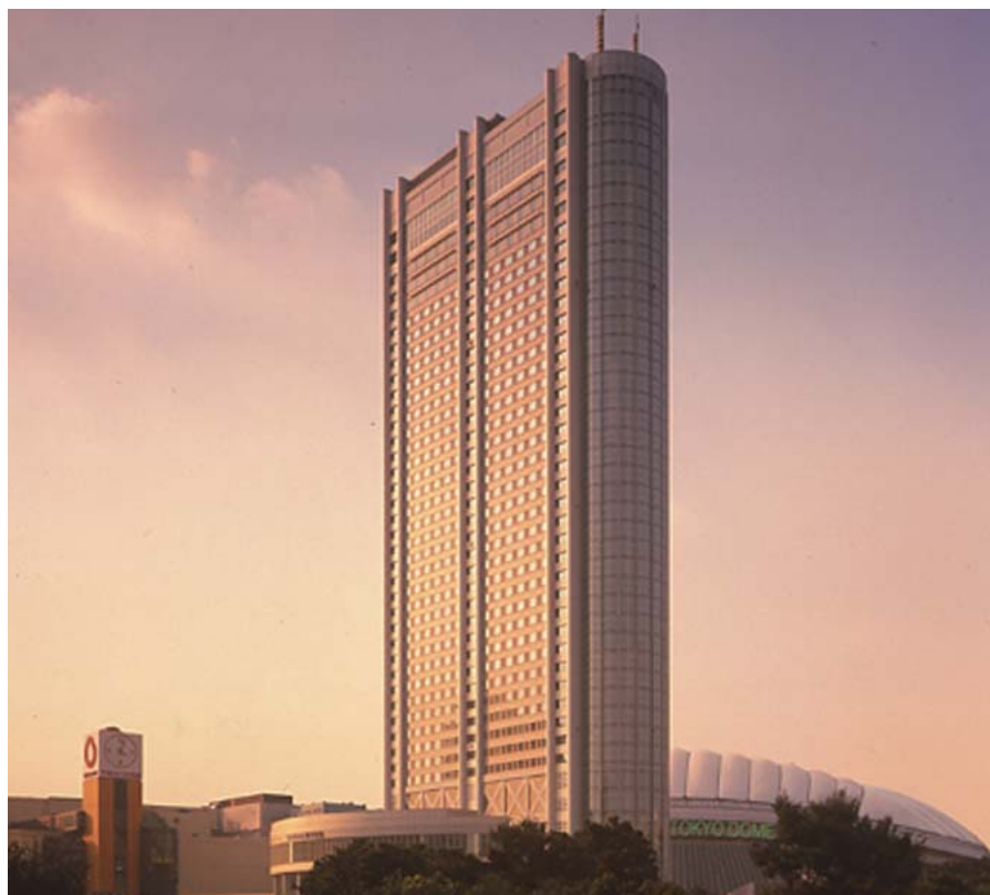
Tokyo Dome Hotel
